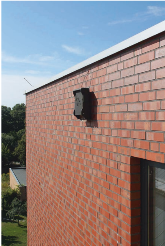
Fig. 14.4 Artificial bat roost on the exterior of the Leibniz Institute for Zoo and Wildlife Research building in Berlin, Germany. Nyctalus noctula use the roost during autumn
