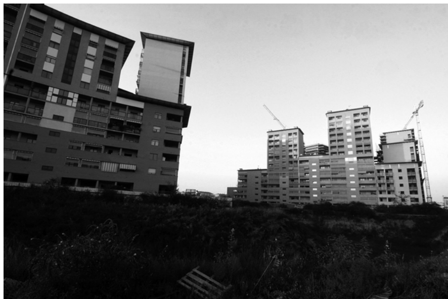
Fig. 6 New housing settlements in Via Cigna (Photo by P. Cingolani)
